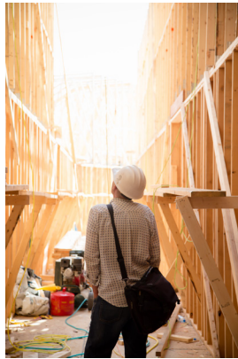
Architect Jude Hallamek reviews recent framing.
